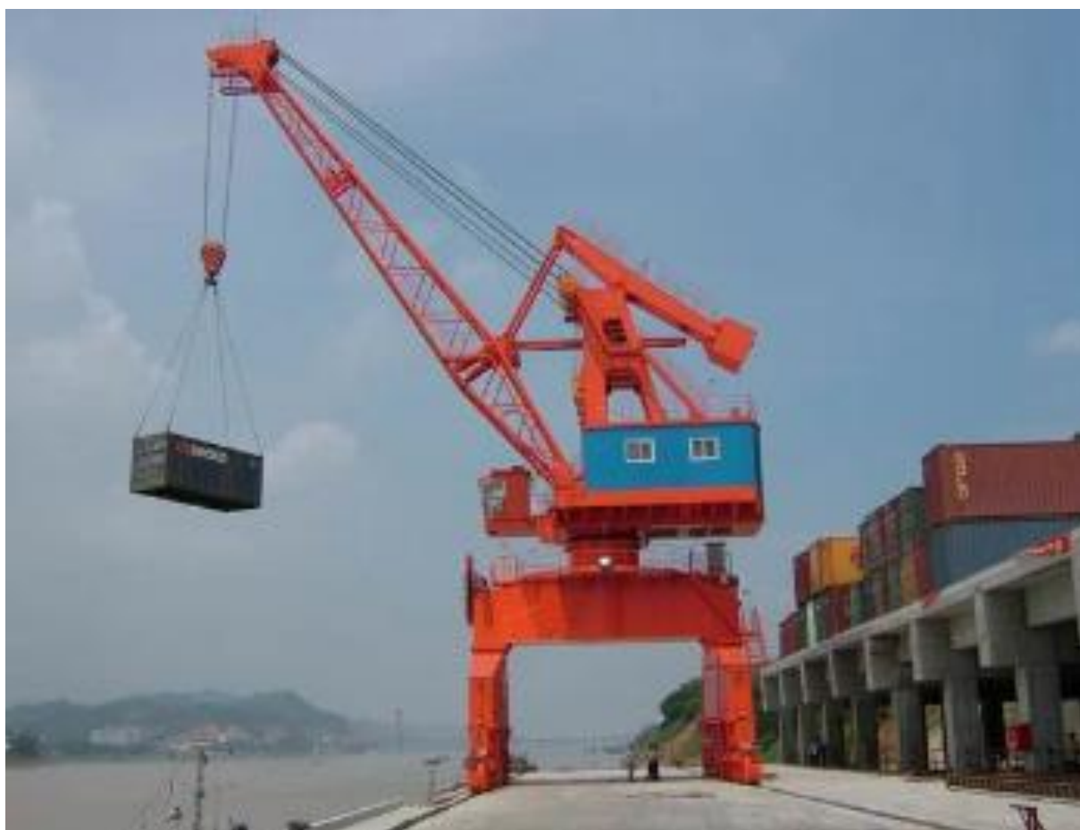
Slika 3.2. Dizalica u luci, Izvor: http://ba.beamcrane.com/port-crane/portal-crane/high-efficient-rail-mounted-portal-crane.html
