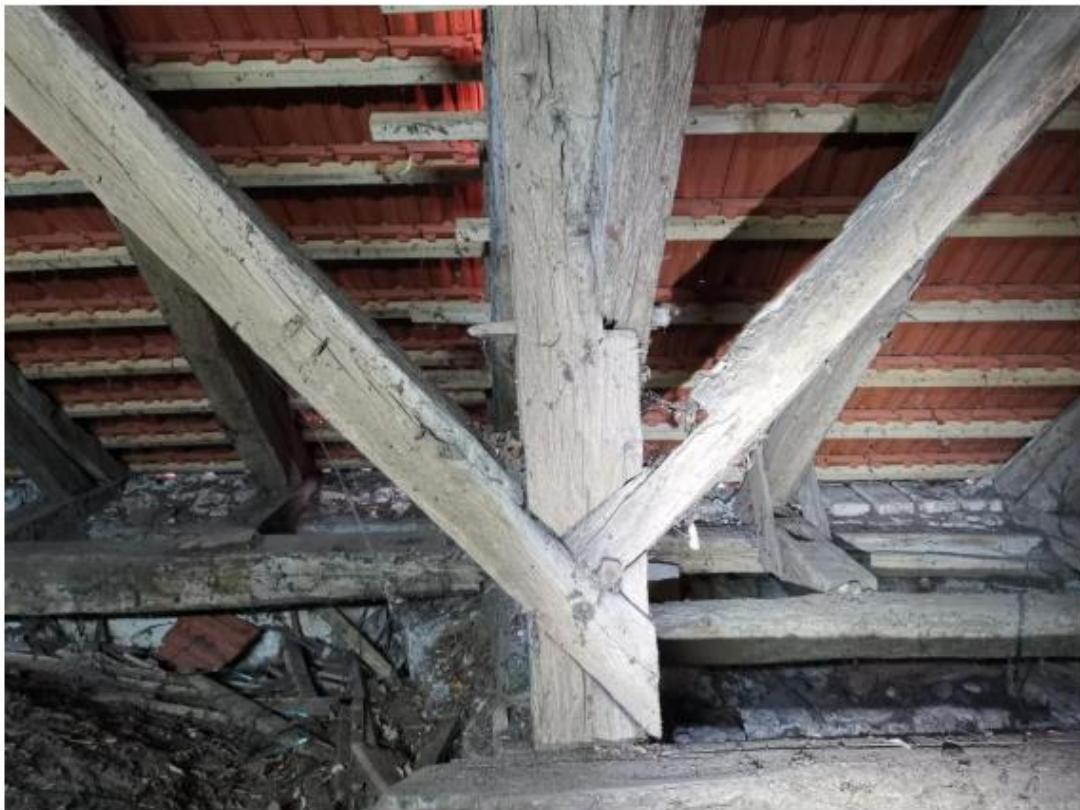
OSLABLJENI SPOJEVI DRVENE KROVNE KONSTRUKCIJE
