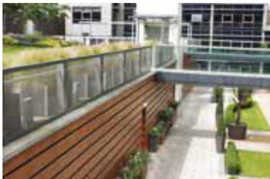
Slika 1 Zeleni krov (GREEN INFRASTRUCTURE Design and Placemaking)
