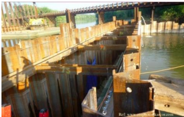
Slika 2.11: Dvozidni koferdam (Izvor: https://www.google.com/search?q=Double-walled+sheet+pile+cofferdams:&sxsrf=ALeKk02Vy9hDIYGgh0iOHEsLu2lloa1SUA:1602017175167&source=lnms&tbm=isch&sa=X&ved=2ahUKEwi0_JiF66DsAhVNPYsKHbb5D0QQ_AUoAXoECA5QAw&biw=798&bih=730#imgrc=3Dte8I2DYJNu2M&imgdii=abjwJk8-bmO5wM )
