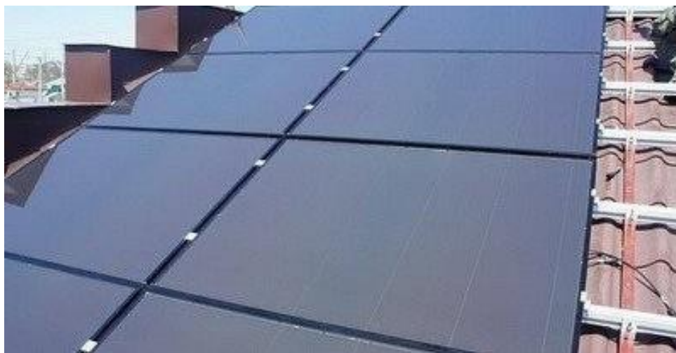
Slika 2.8 amorfni fotonaponski paneli ( https://aquatechn.com/wp-content/uploads/2014/12/solnechnue-batarey4.jpg )
