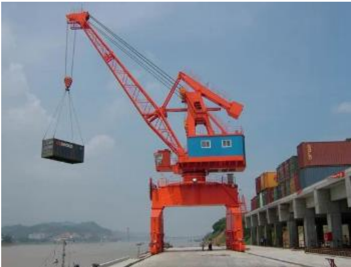
Slika 3.2. Dizalica u luci, Izvor: http://ba.beamcrane.com/port-crane/portal-crane/high-efficient-rail-mounted-portal-crane.html
