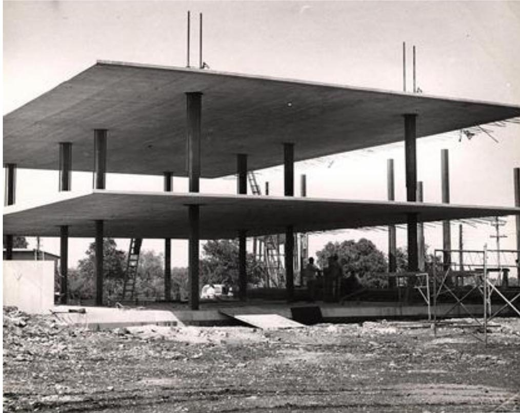
Slika 15: Sistem LIFT SLAB (izvor: <https://theconstructor.org/concrete/lift-slab-construction/6824/>)
