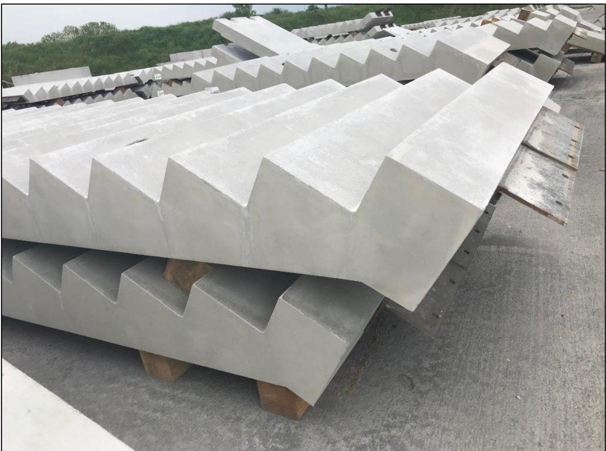
Slika 34: Odlaganje prefabriranih stubišnih krakova (izvor: <https://floodprecast.co.uk/2020/01/benefits-of-using-precast-stairs-with-steel-frame-buildings/>)
