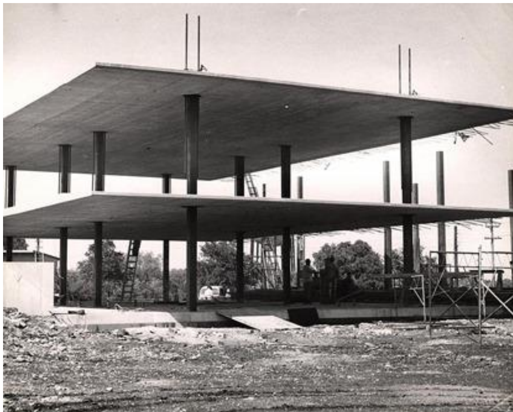
Slika 15: Sistem LIFT SLAB (izvor: https://theconstructor.org/concrete/lift-slab-construction/6824/ )
