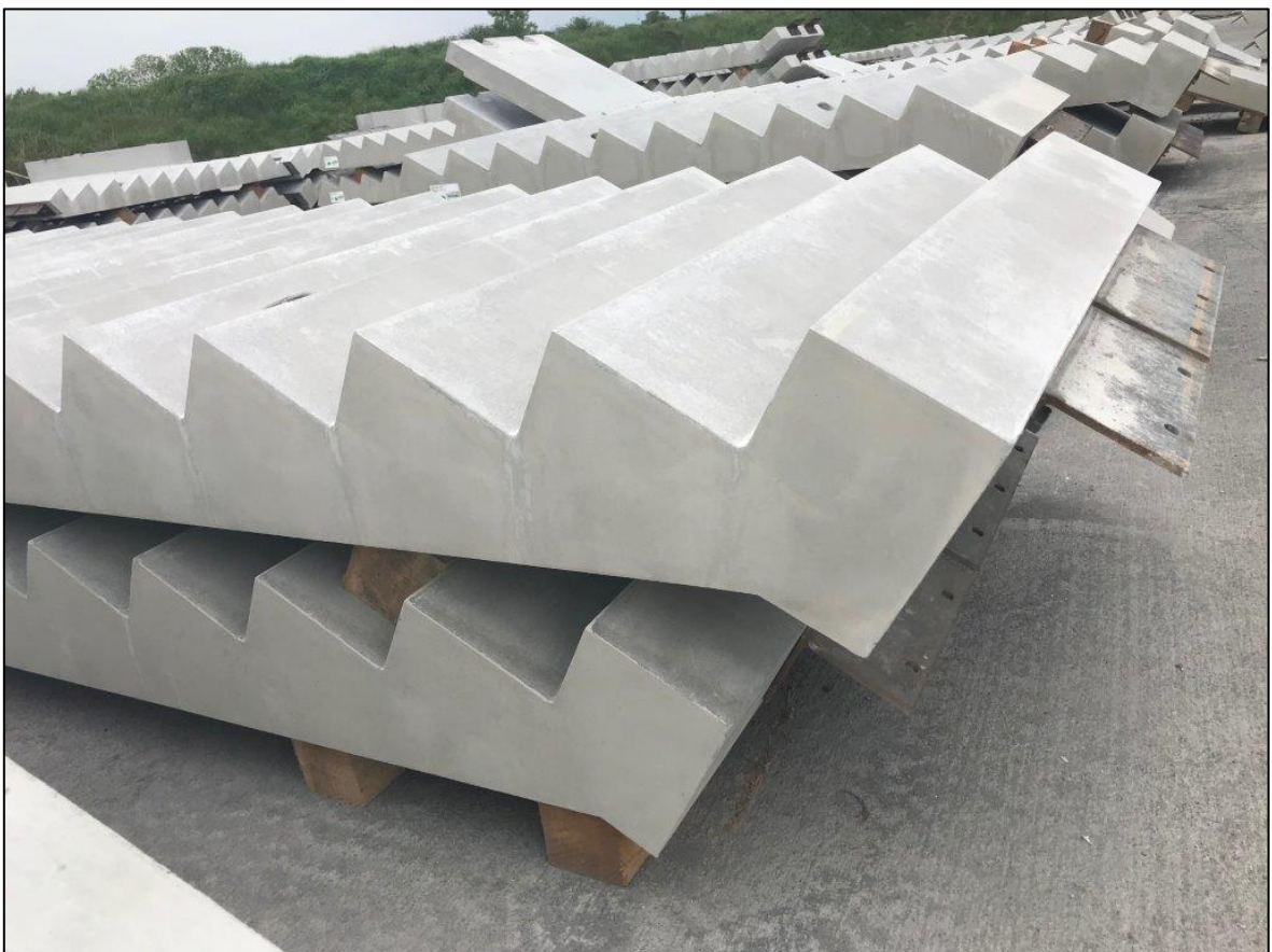
Slika 34: Odlaganje prefabriciranih stubišnih krakova (izvor: https://floodprecast.co.uk/2020/01/benefits-of-using-precast-stairs-with-steel-frame-buildings/ )
