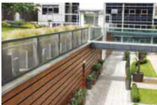
Slika 1 Zeleni krov (GREEN INFRASTRUCTURE Design and Placemaking)
