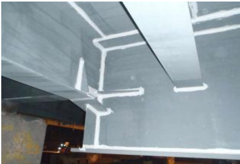
Slika 4. Stripe coating zavara kistom [6]
