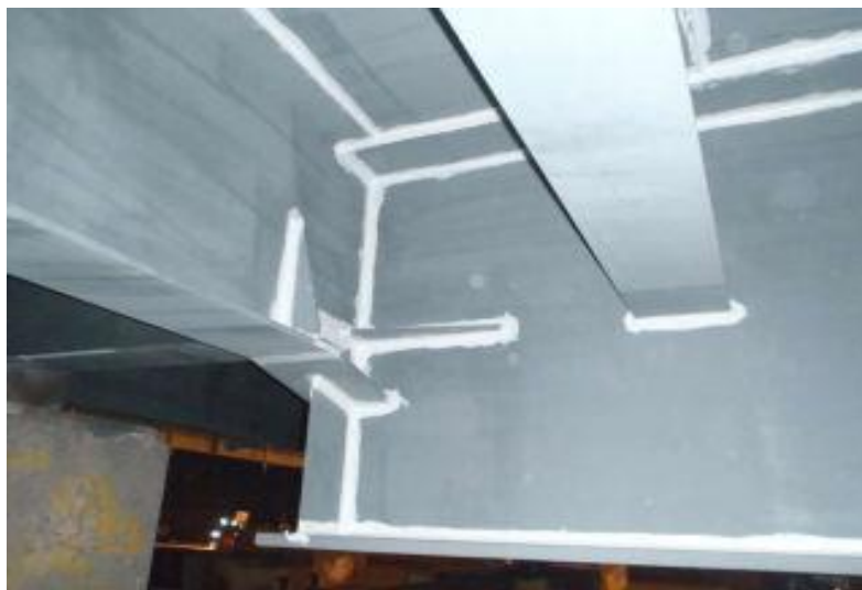
Slika 4. Stripe coating zavara kistom [6]
