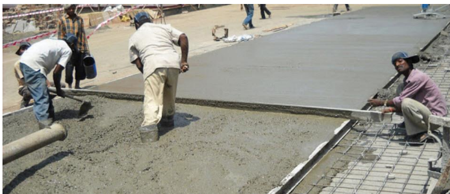
Slika 10. Armirani betonski kolnik (izvor: https://civilatwork.blogspot.com )
