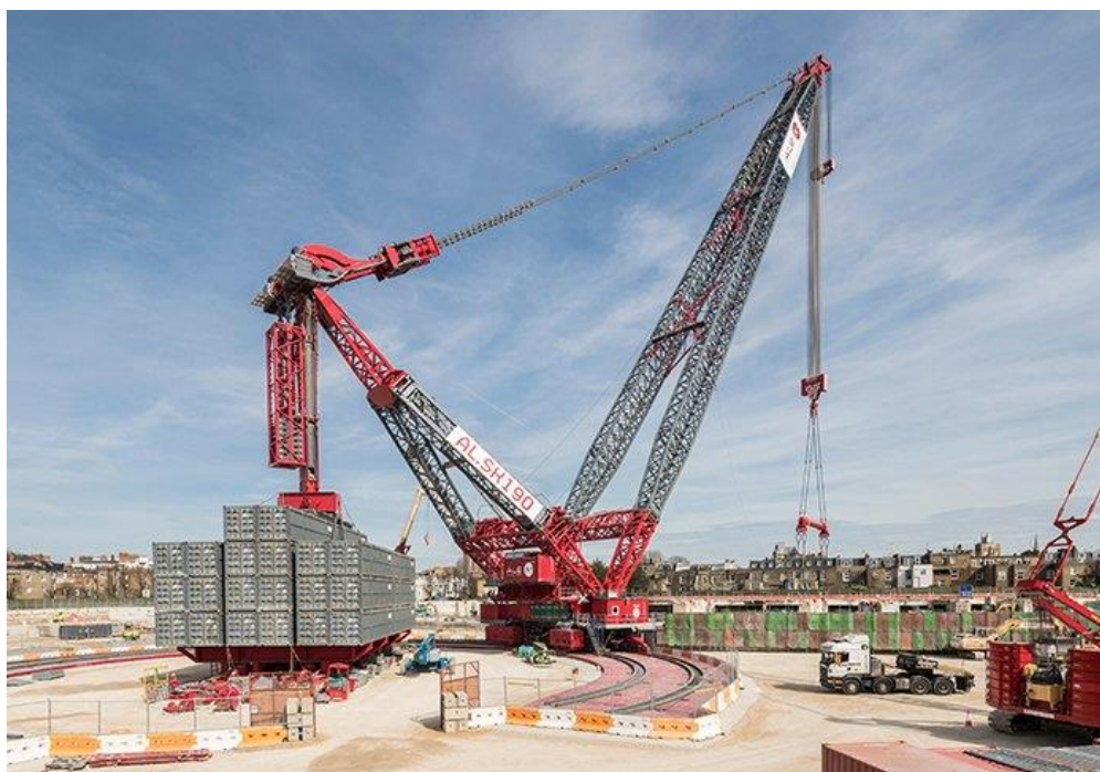
Slika 3.2. Kranška dizalica AL.SK nosivosti 4300 tona na trakastom temeljnom nosaču; Izvor: https://www.ale-heavylift.com/knowledge-centre/case-studies/lifting-portal-beams-with-the-al-sk190-at-earls-court-uk/
