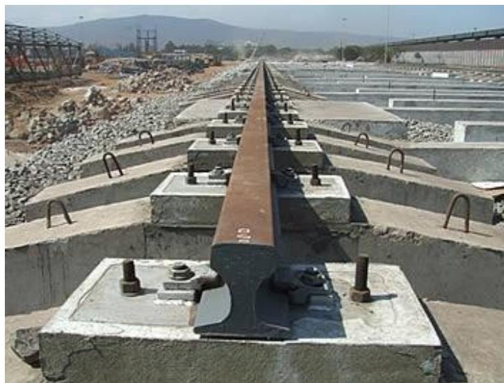
*Slika 3.7. Tračnica kranske staze, Izvor: [http://m.sincholdrail.com/infocrane-rail-installation\\_19583596.html](http://m.sincholdrail.com/infocrane-rail-installation_19583596.html)*
