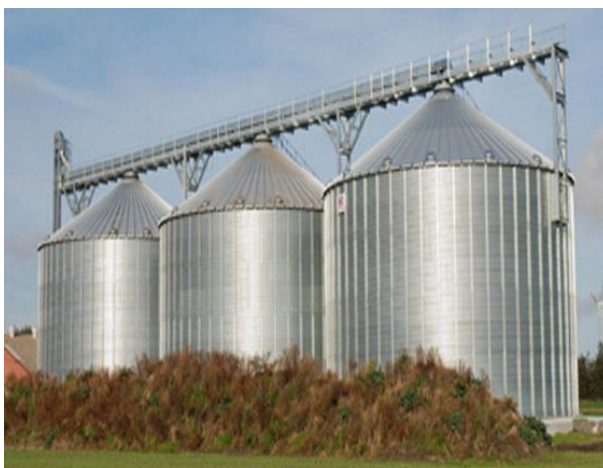
Slika 2.2: Čelični silos (Izvor: http://ba.fdsp-cn.com/wheat-silo-with-competitive-price )
