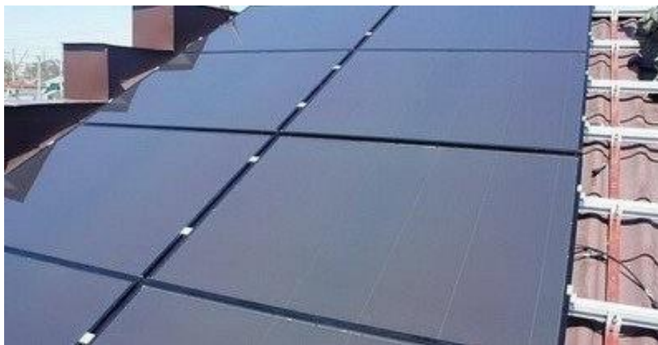
Slika 2.8 amorfni fotonaponski paneli ( https://aquatechn.com/wp-content/uploads/2014/12/solnechnue-batarey4.jpg )
