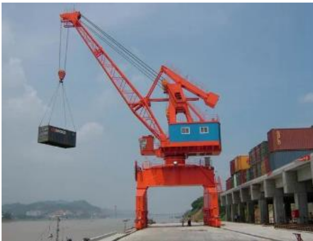
Slika 3.2. Dizalica u luci, Izvor: http://ba.beamcrane.com/port-crane/portal-crane/high-efficient-rail-mounted-portal-crane.html
