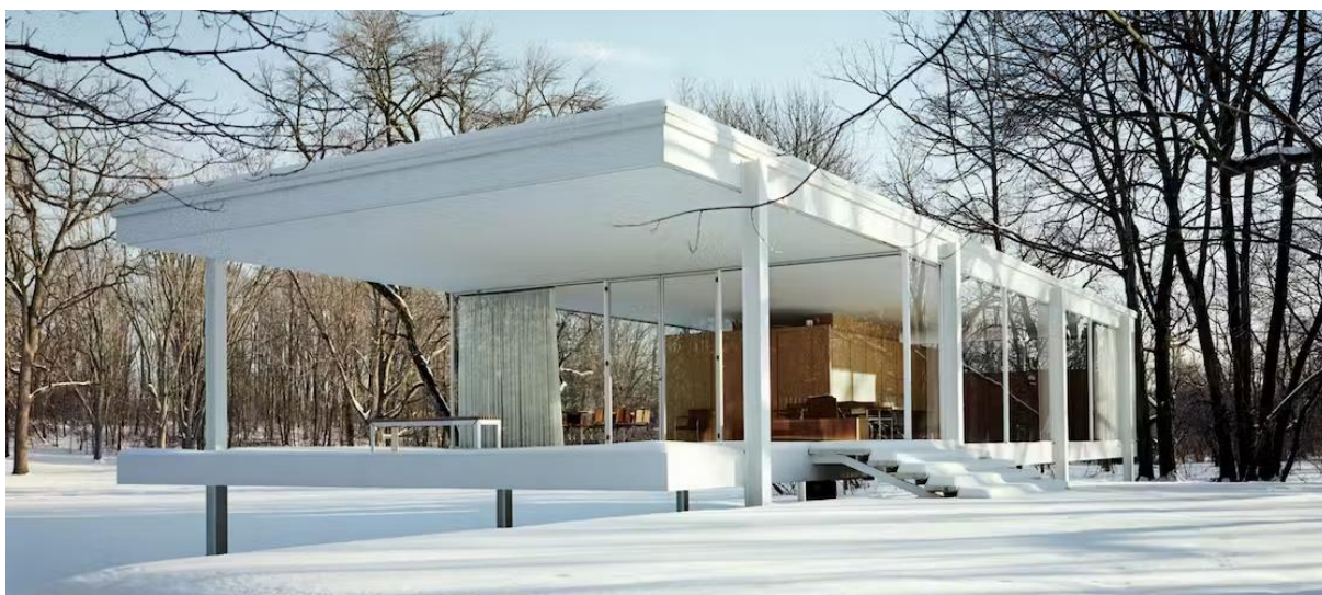
Slika 3-10 Mies van der Rohe, Farnsworth House (1951), Plano, Illinois
