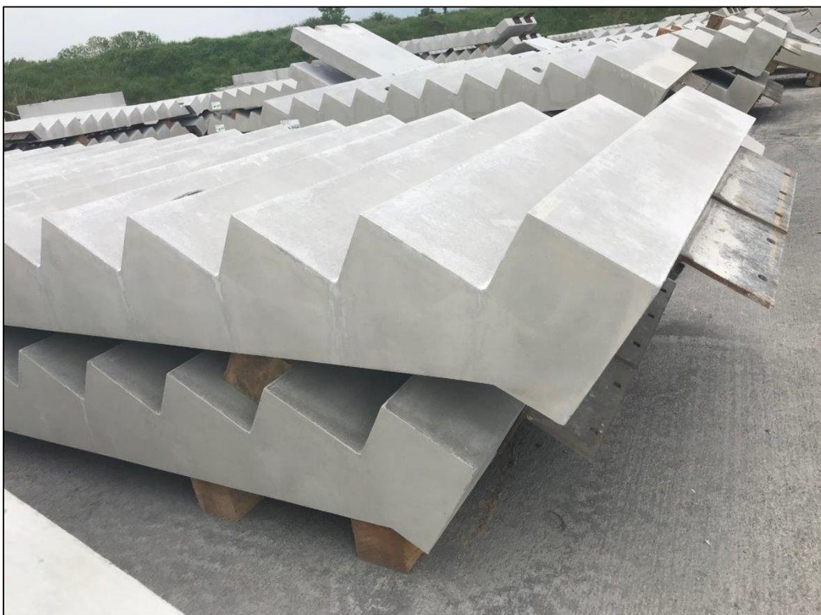
Slika 34: Odlaganje prefabriciranih stubišnih krakova (izvor: <https://floodprecast.co.uk/2020/01/benefits-of-using-precast-stairs-with-steel-frame-buildings/>)
