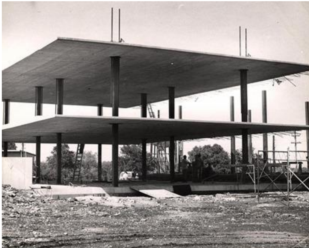
Slika 15: Sistem LIFT SLAB (izvor: https://theconstructor.org/concrete/lift-slab-construction/6824/ )
