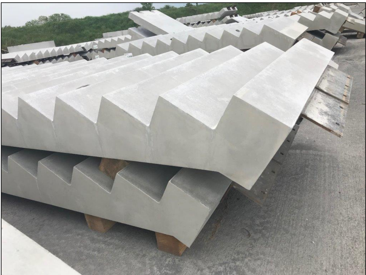
Slika 34: Odlaganje prefabriciranih stubišnih krakova (izvor: https://floodprecast.co.uk/2020/01/benefits-of-using-precast-stairs-with-steel-frame-buildings/ )
