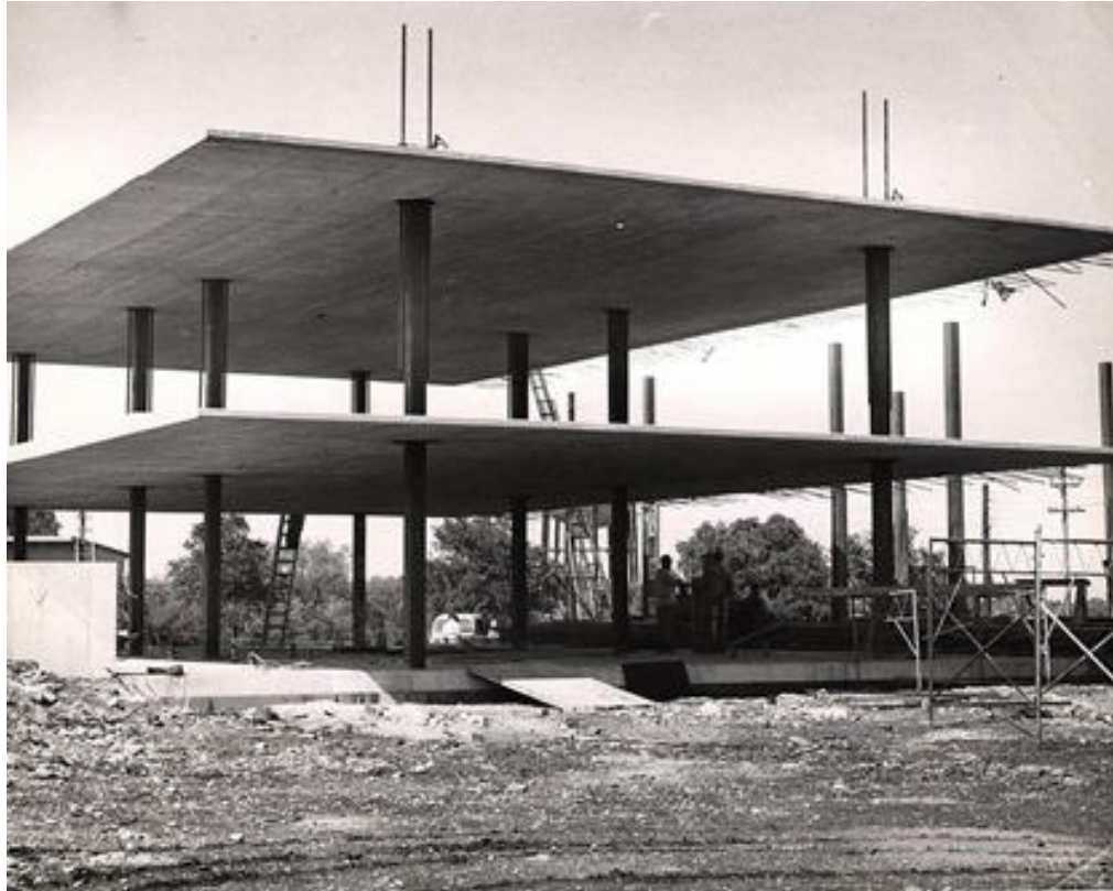
Slika 15: Sistem LIFT SLAB (izvor: https://theconstructor.org/concrete/lift-slab-construction/6824/ )
