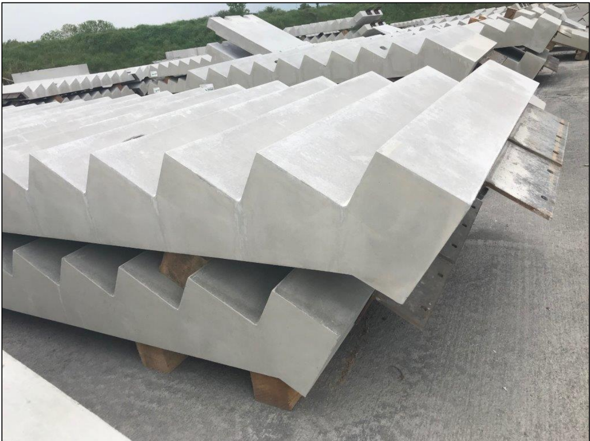
Slika 34: Odlaganje prefabriranih stubišnih krakova (izvor: https://floodprecast.co.uk/2020/01/benefits-of-using-precast-stairs-with-steel-frame-buildings/ )
