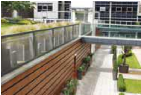
Slika 1 Zeleni krov (GREEN INFRASTRUCTURE Design and Placemaking)
