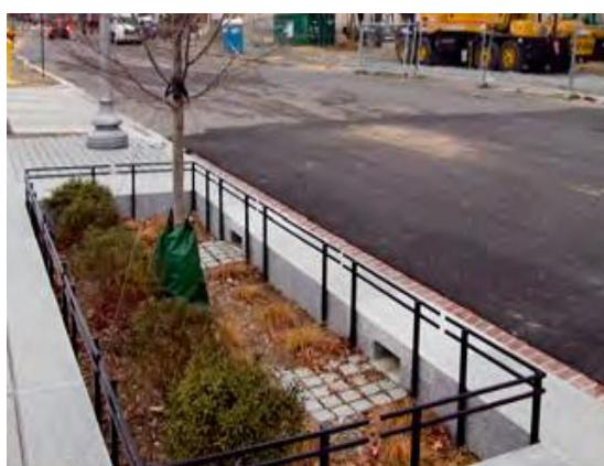
*Slika 13 Infiltracijski jarak (RPA - 9 Ways to Make Green Infrastructure Work)*
